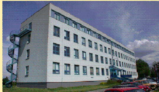
Air Navigation Services (ANS) Hotel and Training Center
